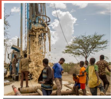
Drilling a groundwater borehole in Ethiopia (© UNICEF Ethiopia 2016 / Ayene / Flickr)
